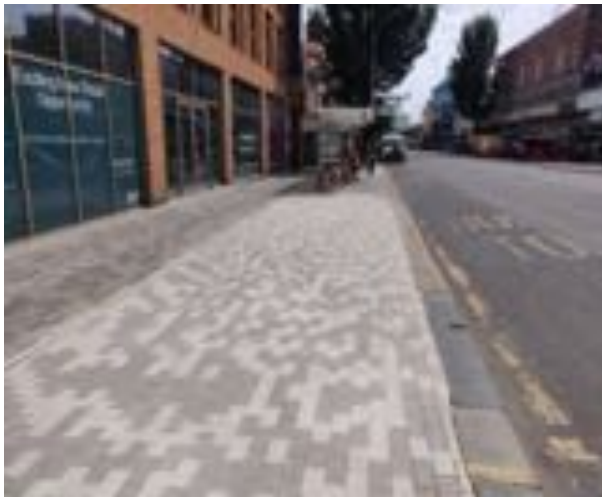
Photo of London Road where 10 bicycle racks should be
