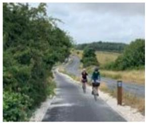
The shared use path along the Ditchling Road, between Woodbourne Avenue and Old Boat Corner (where Stanmer Woods begin) has been resurfaced, with asphalt replacing the loose gravel that was frequently eroded by rain and overgrown. The new cycling, wheeling and walking path is now a reasonable 3.5 metres wide, which reduces potential conflicts with other users, although brambles are beginning to intrude.
